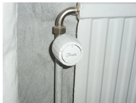
Figure 3. The design of a thermostatic radiator valve showing a range of 0–6 levels. (Source: Author's collection.)
