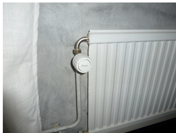
Figure 1. A typical radiator fitted with a thermostatic radiator valve. (Source: Author's collection.)
